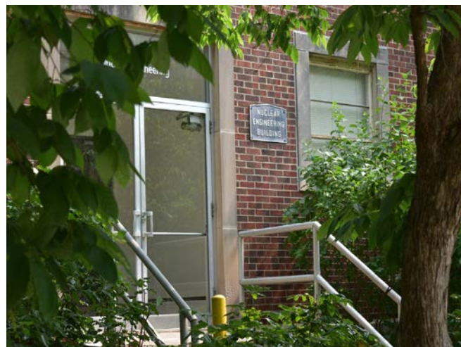
The previous Nuclear Engineering building
