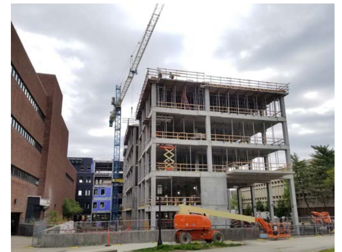
Construction progress is made in early fall 2021
